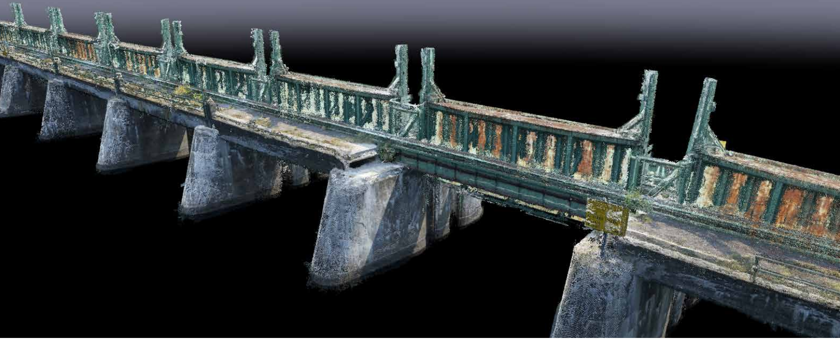
Using highly accurate data collected using a microdrones UAS, a preservation agency was able to create a 3-dimensional model of the Fryer Dam that engineers could use when drafting their proposals.
